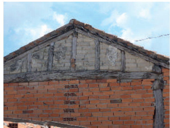
Fig. 1 Images of recurring interventions using industrial brick in the restoration of adobe walls. Left: Congosto de Valdavia (Palencia); Right: Arroyo de Cuéllar (Segovia)
